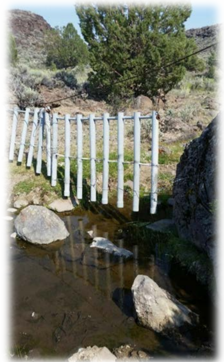
PVC piping that protects creek portion of enclosure from entry (Continued on next page)
