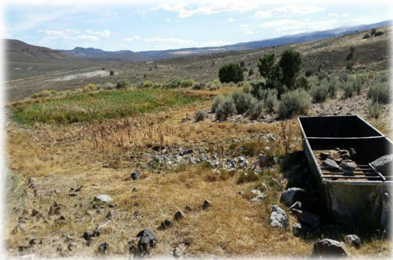
Developed Spring System and Trough Needing Repair
